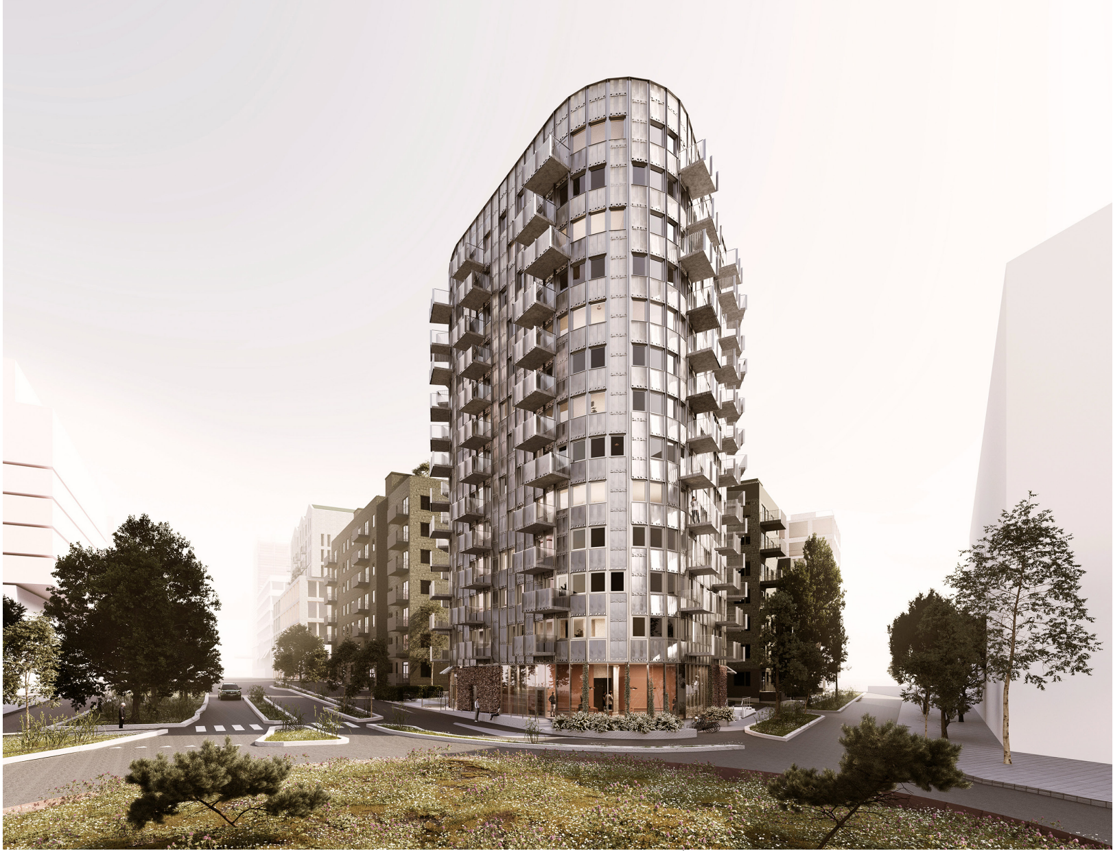
Droppen, a residential building in Malmö, Sweden, found a novel use for heat exchanger plates.
