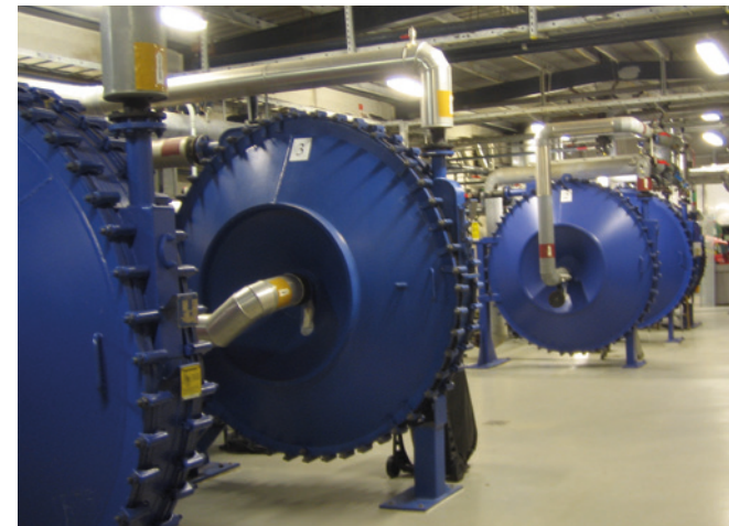
4 of 5 Alfa Laval spiral heat exchangers installed in the pre-heating section.
