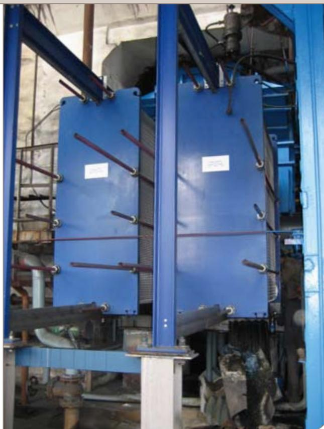
Compared to shell-and-tube, the Alfa Laval solution facilitates maintenance. AlfaCond is easy to open for mechanical cleaning. Chemical cleaning, too, is facilitated by the low hold-up volume of the compact AlfaCond condenser. Even more importantly, Avdeevka no longer needs to shut down the turbine every time a condenser tube is leaking, thus reducing expensive downtime.
