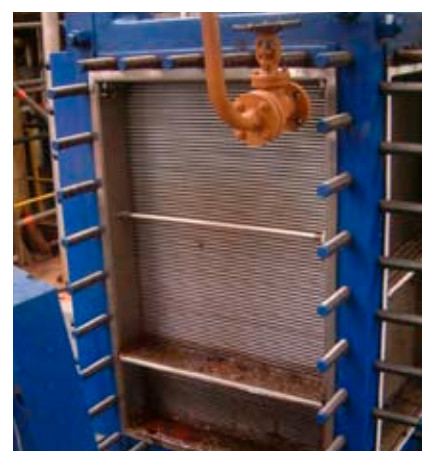
Photo showing before and after high-pressure water-jet cleaning of the cooling water circuit of a Compabloc operating as condenser in the solvent recovery part of a paraffin removal plant in Europe.
