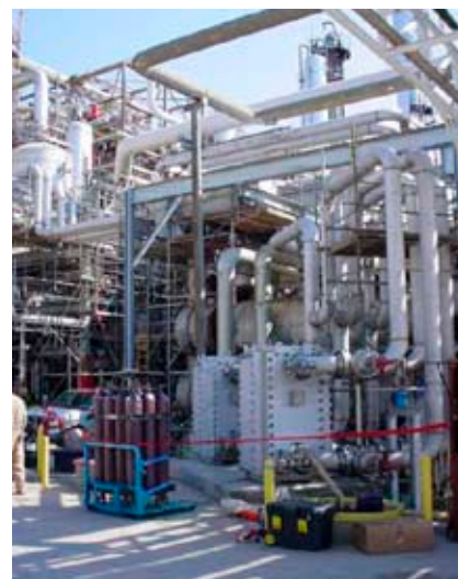
Two Compablocs preheating crude since 2004 in a North American refinery.
