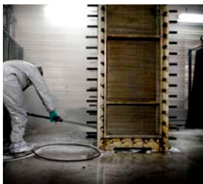
This means the hydro-jet passes through the heat exchanger when the nozzle is tilted in 45 degree angle.
